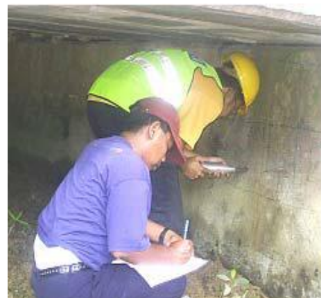
Fig 13: Rebound hammer test conducted on selected abutment
