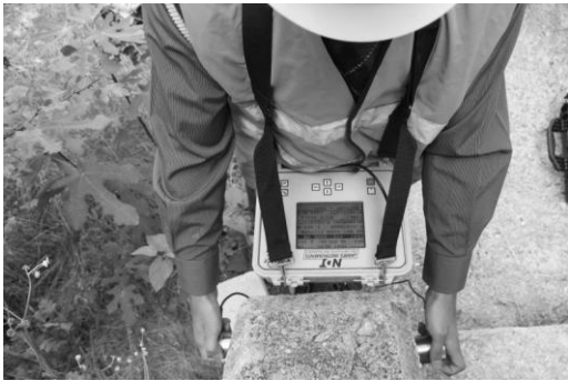
Fig 20: Application of ultrasound pulse velocity device on a concrete bridge wing wall.
